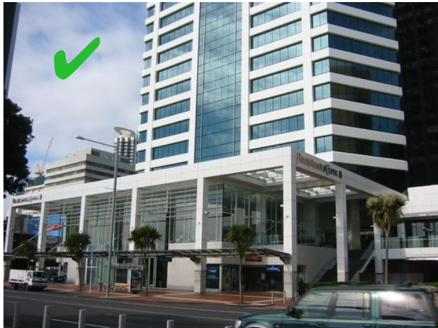
8. Undercover car-parking not located on street frontage
